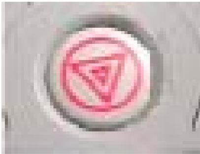
button cuts power to the magnet room and removes electrical power to all components of the system other than the static magnetic field and the Magnet Shutdown Unit. (2) Evacuate the subject. (3) Pull the fire alarm and call Campus **911**. (4) Use the fire extinguishers to
